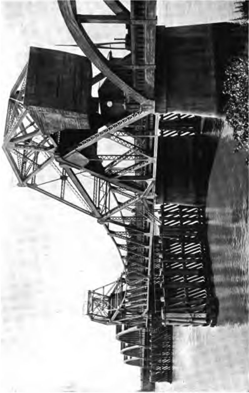
Bascule bridge over Sacramento River at Rio Vista. This bridge supplies a cross-state connection by way of Rio Vista and Suisun.
